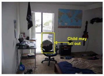
The window adjacent to the entry doors of many units are potential safety hazards as the glazing in the windows did not appear to be tempered glass. Windows within 24" of the strike/closing side of a door are to be tempered glass for safety as a locked out tenant or burglar may attempt to break the window to gain access. Replacement with tempered glass is advised. Consult a licensed glazing contractor for further evaluation.
