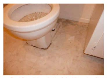
The toilet tank is cracked, and should be replaced before it breaks completely and causes water damage.
